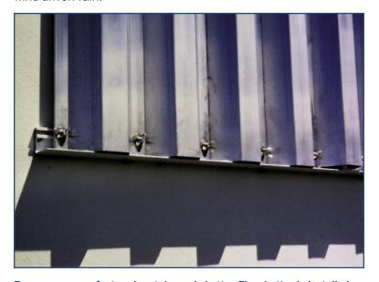
Temporary, manufactured metal panel shutter. The shutter is installed in a track permanently mounted above and below the window frame. The shutter is placed in the track and secured with wing nuts to studs mounted on the track. This type of shutter is effective and quickly installed, and the wing nut and stud system provides a secure anchoring method.
