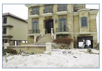
Large solid stairs such as these block flow under a building and are a violation of NFIP free-of-obstruction requirements.
