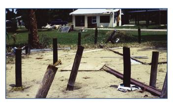
Insufficient pile embedment and failure of connections at tops of piles allowed elevated building to be floated off its foundation.
