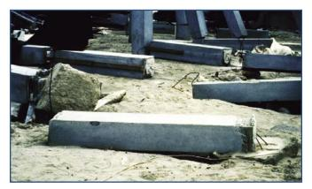
Pier (column) failures: footings undermined and columns separated from footings.
