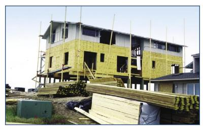
Figure 4 Vertical addition to a home damaged by Hurricane Fran. Preexisting 1-story home became the second story of a home elevated to meet new foundation and floor elevation requirements.
