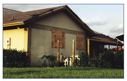
Plywood panels are a cost-effective means of protection.
