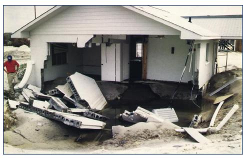
Building failure caused by undermining of slab-on-grade foundation during Hurricane Fran.
