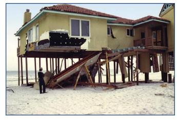
Pile failures led to collapse of floor of elevated building.
