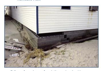
Failure of crawlspace foundation undermined by scour.
